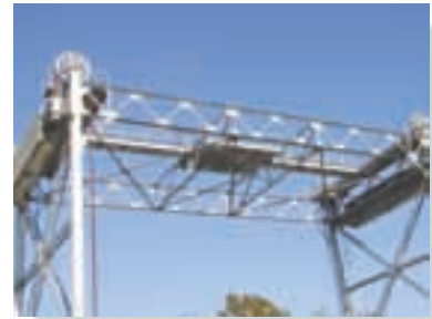
The use of metal gusset plates in the construction of these Warren trusses is clearly evident. (© Russell C. Hibbeler)
