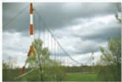
The cable and suspenders are used to support the uniform load of a gas pipe which crosses the river. (© Russell C. Hibbeler)
