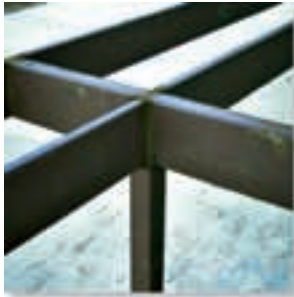
The floor beams of this building are welded together and thus form fixed connections. (10) (© Russell C. Hibbeler)
