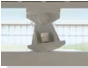
The rocker support for this bridge girder allows horizontal movement so the bridge is free to expand and contract due to a change in temperature. (4) (© Russell C. Hibbeler)
