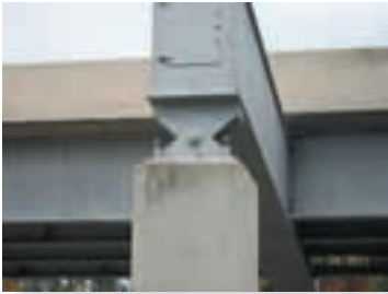
Typical pin support for a beam. (8) (© Russell C. Hibbeler)
