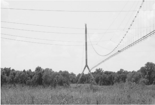
Cables support their loads in tension.
