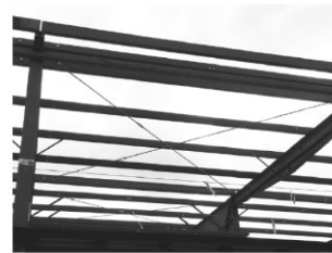
Tie rods used for wind bracing.
