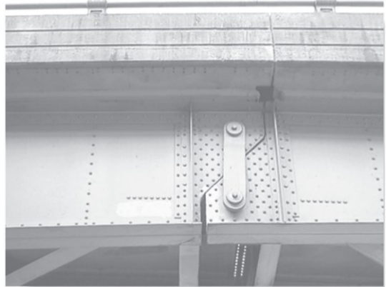
The short link is used to connect the two girders of the highway bridge and allow for thermal expansion of the deck.
