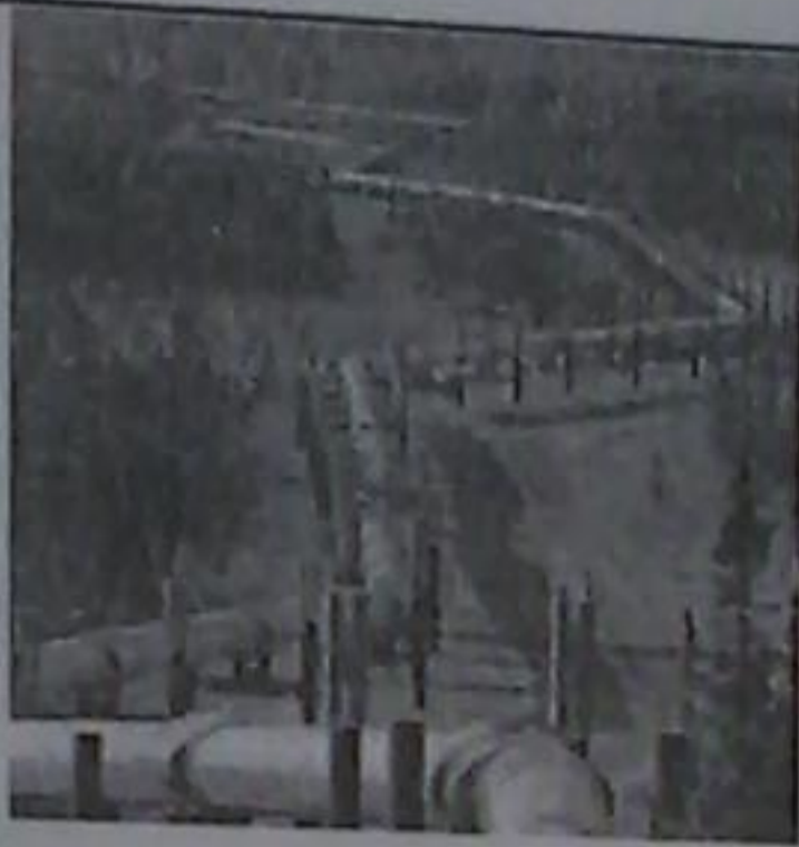
The Alaskan pipeline, a significant accomplishment of the engineering profession, transports oil 1286 km across the state of Alaska. The pipe diameter is 1.2 m, and the 44 pumps are used to drive the flow
