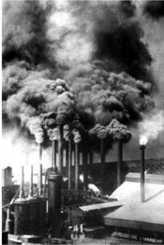
Sign of prosperity in Pittsburgh in 1906 (Source: Carnegie Library of Pittsburgh)
