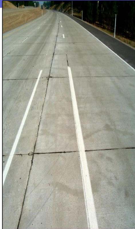
Rigid (concrete) pavement
