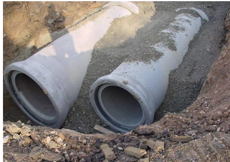
New construction of a separated sewer system in Germany.
