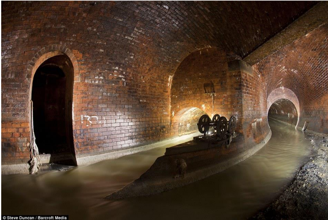
A brick-built sewer chamber under Clapham High Street in south London
