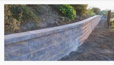
Retaining Wall Contractor & Repair ... 2020landtree.com
