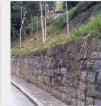
Retaining wall - Wikipedia en.wikipedia.org
