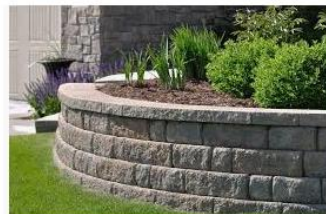
Retaining Walls Melbourne - Blocks ... everlastservices.com.au
