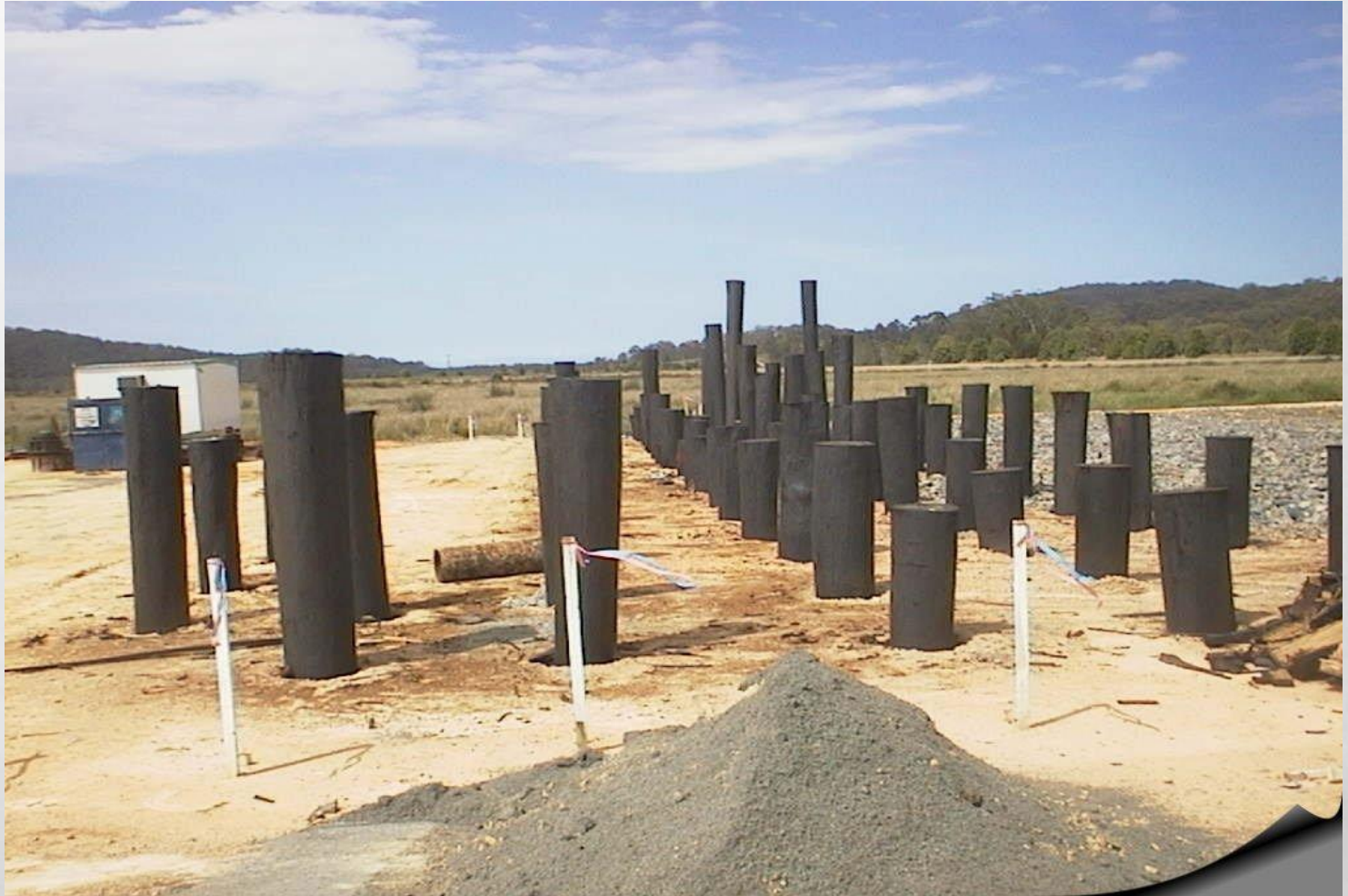
Driven timber piles, Pacific Highway
