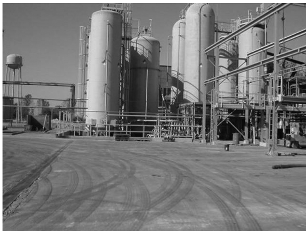
FIGURE 15.5 Hazardous waste storage tanks. These tanks can store over 350,000 gal of hazardous waste.
