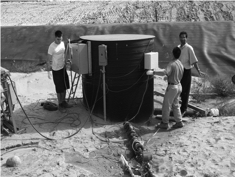
FIGURE 10.26 Landfill sump installation. (Reproduced with kind permission of Environmental Research and Education Foundation, Bioreactor Landfill Project Northern Oaks Landfill , 2002, Available from: http://www.erefndn.org/rpts_summary_ordrs/northern Oaks.htm .)
