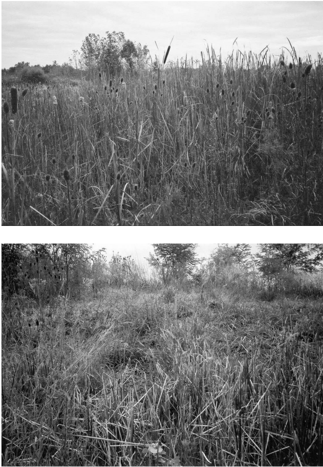
FIGURE 10.1 Landfill operated and closed prior to the enactment of RCRA regulations. Subsidence has occurred, creating a toxic wetland. Leachate is exiting freely from the sides of the landfill.
