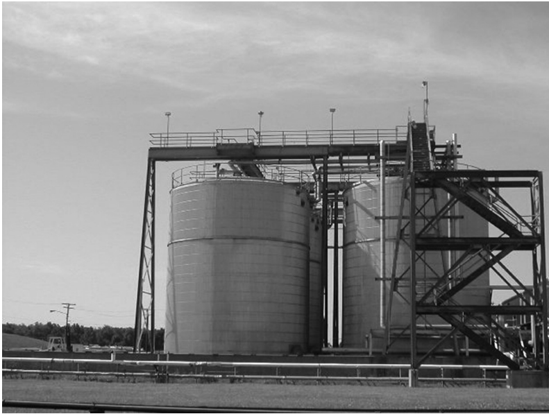
FIGURE 17.8 Tanks for storage and blending of liquid hazardous wastes.
