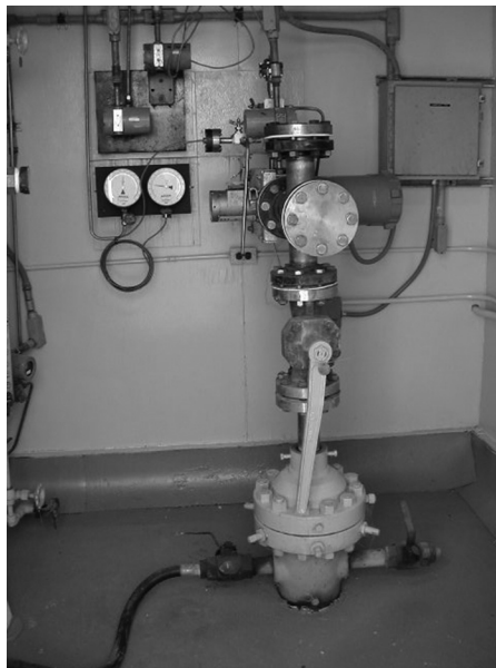
FIGURE 17.9 Well head at deep-well injection facility.
