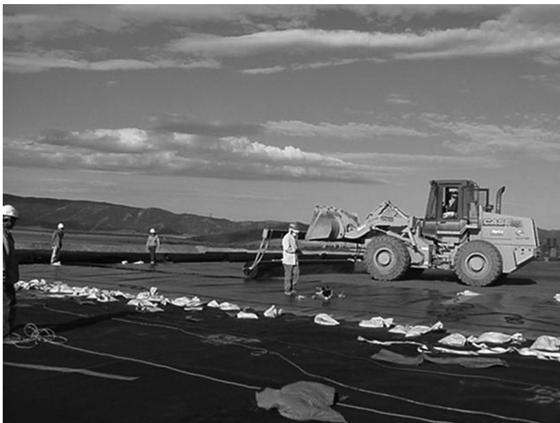
FIGURE 10.4 Geomembrane material being installed at a land disposal facility. (From EPA.gov.)
