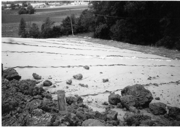
FIGURE 10.30 Landfill cap under construction showing overlapping sheets of geomembrane cap.
