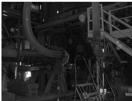
FIGURE 15.8 Injection ports for the introduction of liquid hazardous wastes to a rotary kiln.
