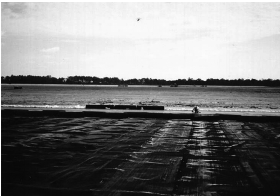
FIGURE 17.2 Geosynthetic landfill liner being installed. (Reproduced with kind permission of Tenax, Baltimore, MD, Available from: http://www.tenax.net/geosynthetics/products/geocomposite-mdp.htm .)
