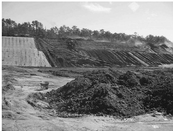
FIGURE 10.3 Installation of a layer of low-permeability clay. The clay is spread in two lifts and then rolled. (Reproduced with kind permission of ISWM Operations, Landfill , No date, Available from: http://www.townofbourne.com/Departments/PUBLICWORKS/IntegratedSolidWasteManagment/ISWMOperations/tabid/333/Default.aspx .)
