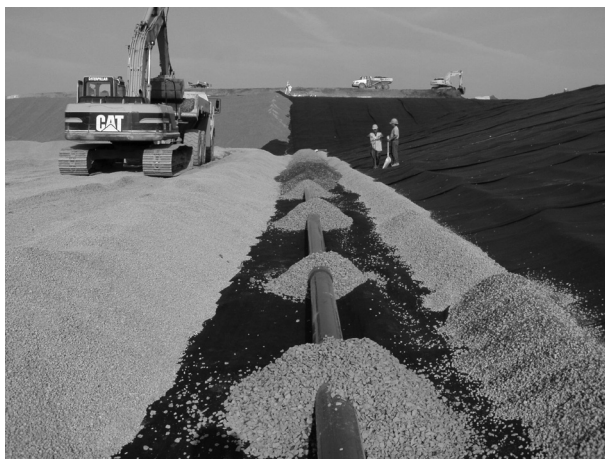
FIGURE 17.4 Photograph of an LCR system. (From Seneca Meadows Landfill, Solid Waste Management , 2014. Available from: http://www.senecameadows.com/facilities_waste.php . Reproduced with kind permission from Duprey Video Productions, Waterloo, NY.)
