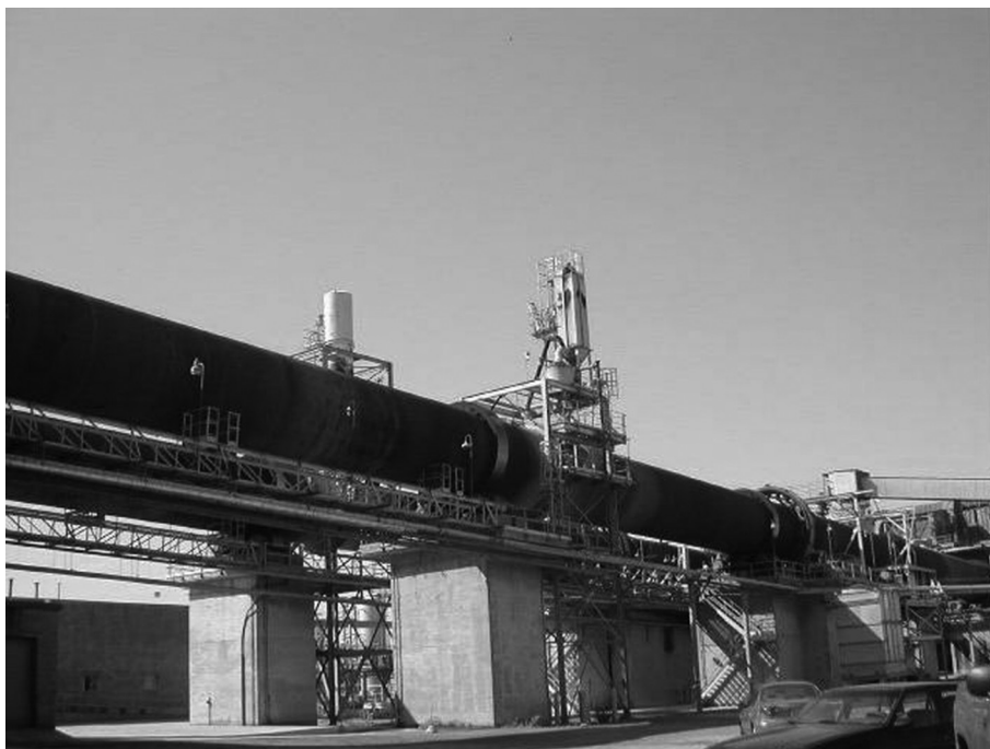
FIGURE 15.11 Dual cement kilns, each measuring 450 ft in length with a 1 in. steel shell lined with 9–12 in. of firebrick. This facility handles 25 million gal of hazardous waste per year.
