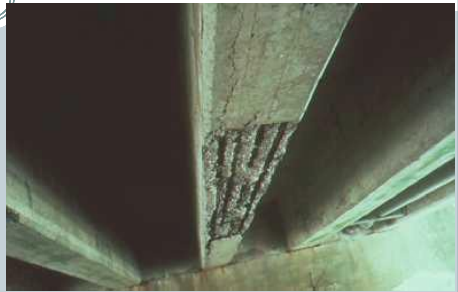
✓ Delamination of A Concrete Beam
