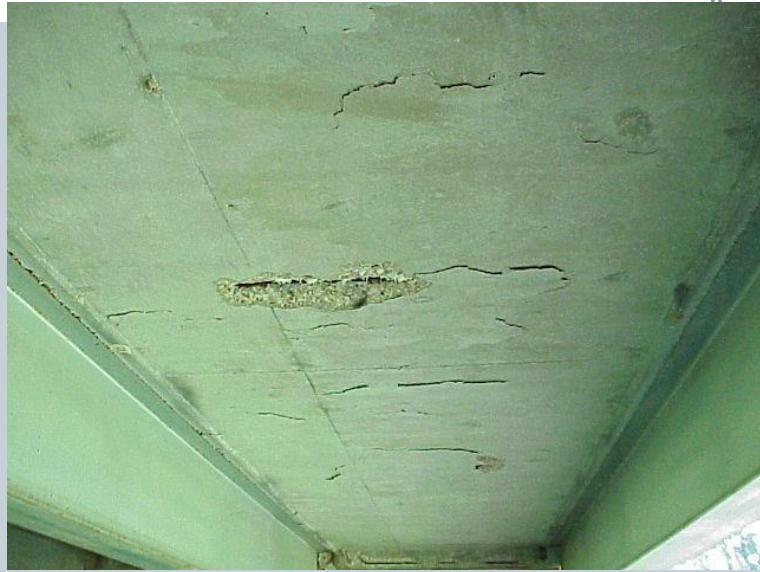
✓ Spalling
