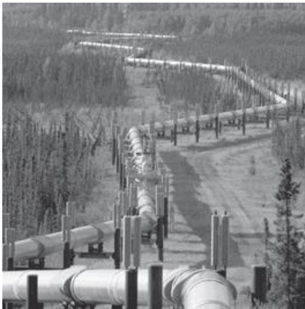
*The Alaskan pipeline, a significant accomplishment of the engineering profession, transports oil 1286 km across the state of Alaska. The pipe diameter is 1.2 m, and the 44 pumps are used to drive the flow*
