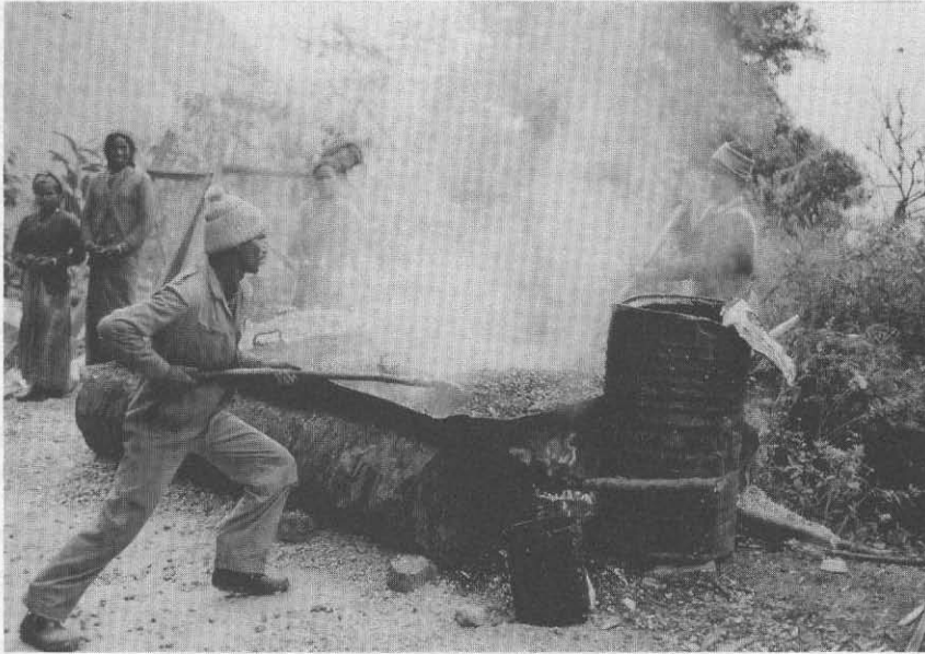
Figure 19.4 Hand-mixing hot asphalt in India.
