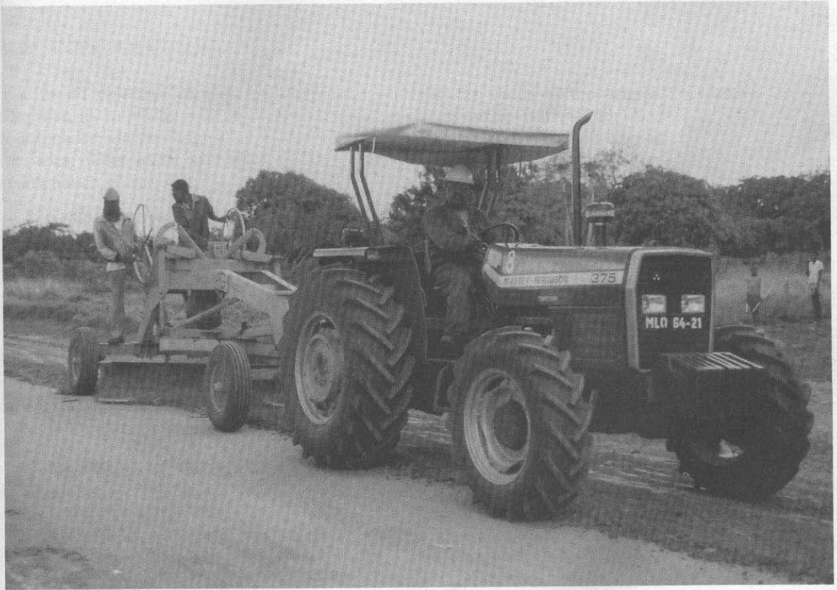
Grading of gravel roads in Mozambique. (Photo by Bent Thagesen)
