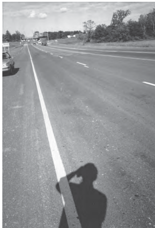
FIGURE 3.32 Example of bleeding in flexible pavement.
