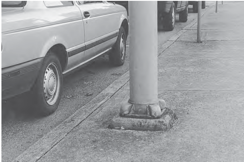
FIGURE 7.73 Flange-type steel base.
