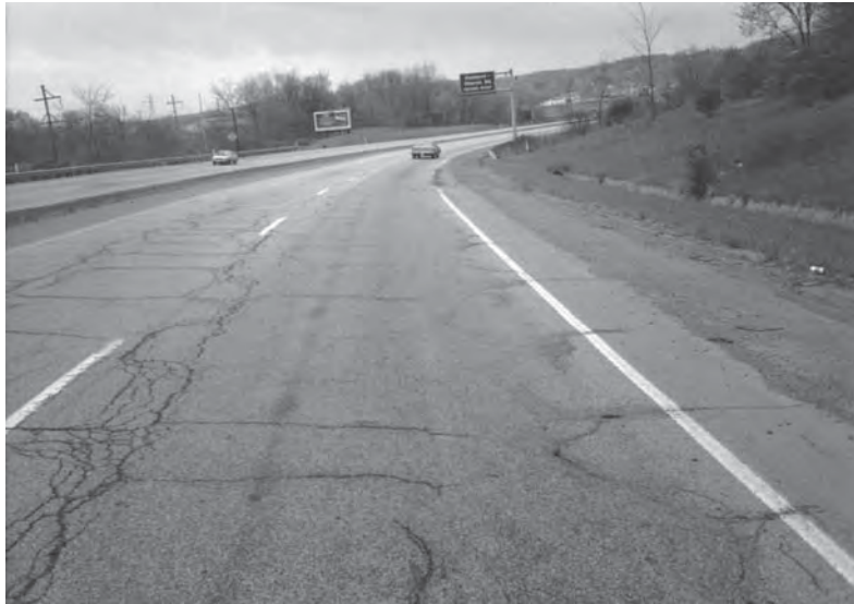
FIGURE 3.38 Example of block cracking in flexible pavement.
