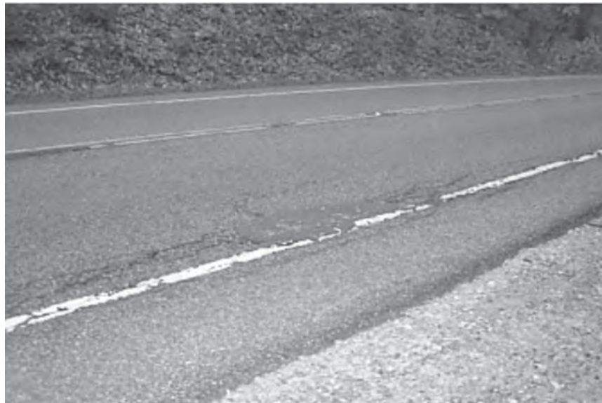
FIGURE 3.57 Localized wheel track and edge cracking.
