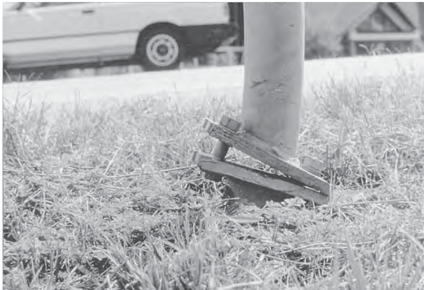
FIGURE 7.17 Loose slip base caused by vibration.
