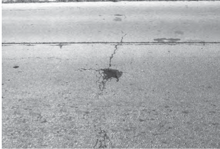
FIGURE 3.33 Example of small pothole in flexible pavement.
