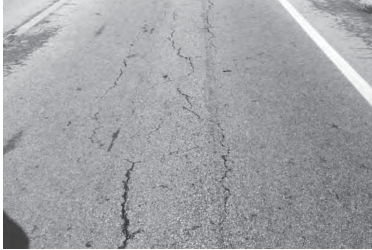
FIGURE 3.36 Example of longitudinal cracking in flexible pavement.
