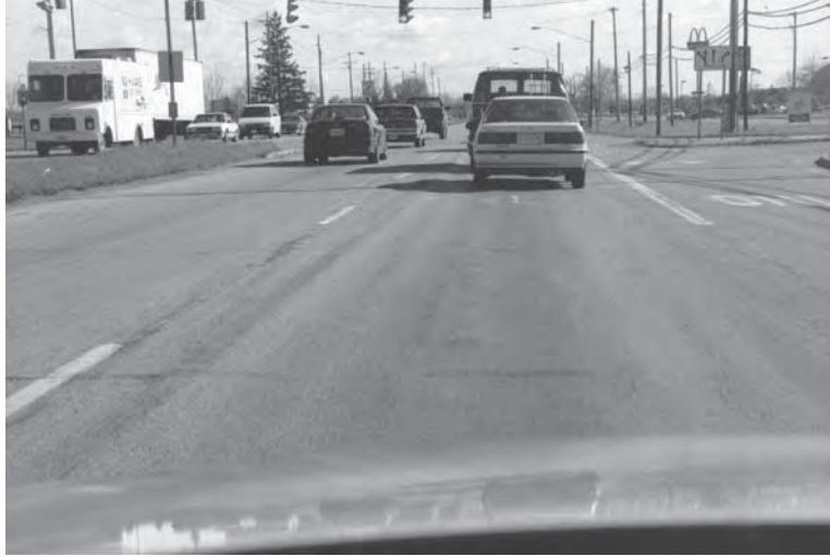
FIGURE 3.34 Example of rutting in flexible pavement.
