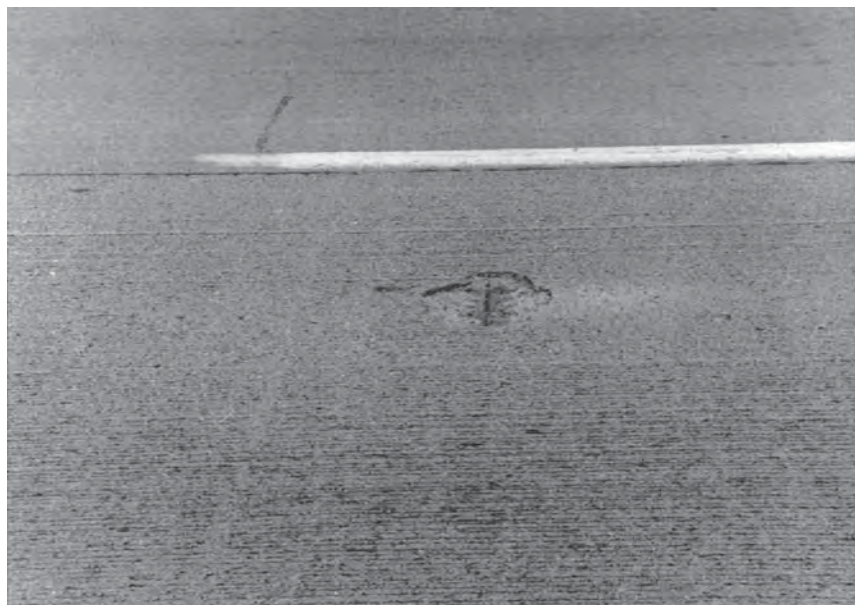
FIGURE 3.23 Example of popout in jointed rigid pavement.
