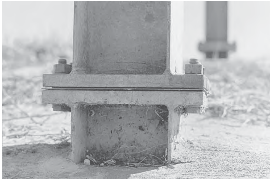
FIGURE 7.25 Installation of horizontal slip base.
