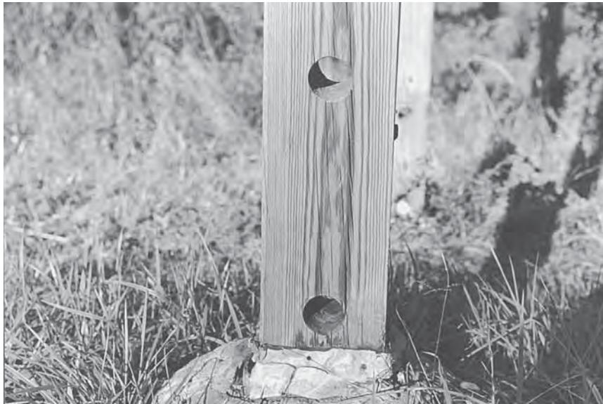
FIGURE 7.46 Weakened wooden post for multiple supports.
