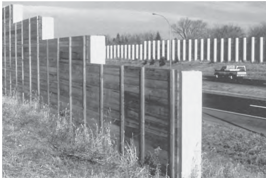
FIGURE 9.5 Timber noise barrier with concrete posts showing effect of contrasting hues.
