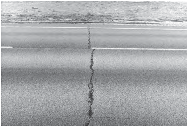
FIGURE 3.37 Example of transverse cracking in flexible pavement.
