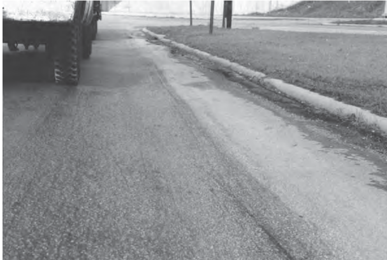
FIGURE 3.35 Example of corrugations in flexible pavement.
