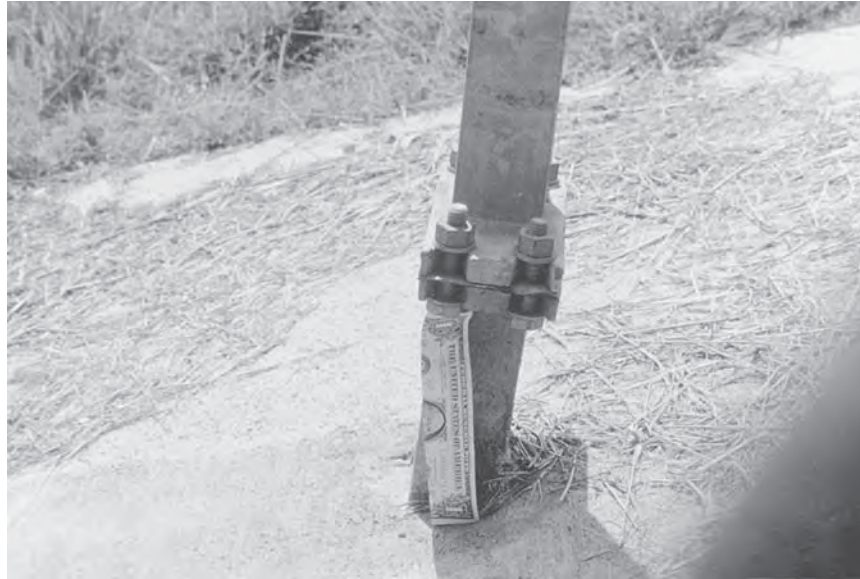
FIGURE 7.37 Improper installation of slip base anchor piece.
