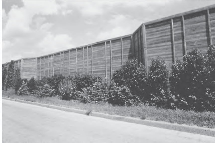
FIGURE 9.4 Timber noise barrier with buttress-type alignment.
