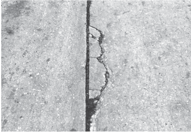
FIGURE 3.25 Example of joint spalling in rigid pavement.
