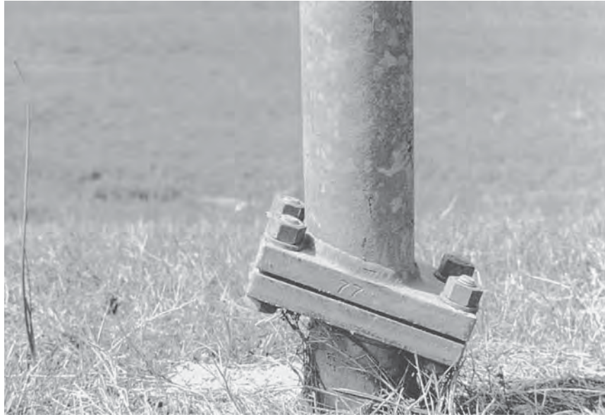
FIGURE 7.18 Installation of unidirectional slip base.
