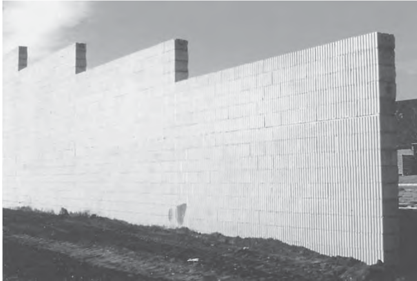
FIGURE 9.2 Concrete-block noise barrier with vertical groove treatment, stepped in height.
