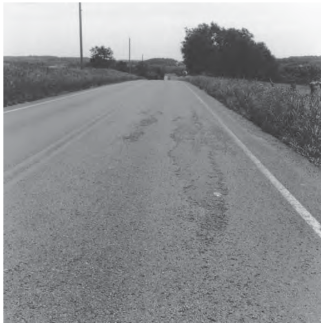
FIGURE 3.31 Example of raveling in flexible pavement.
