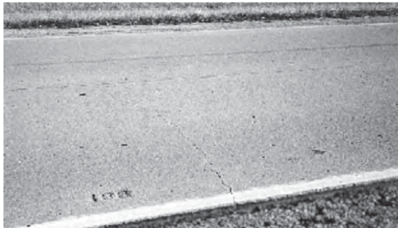
FIGURE 3.55 Hairline crack in rigid pavement.
