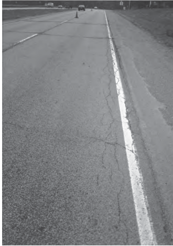
FIGURE 3.40 Example of edge cracking in flexible pavement.
