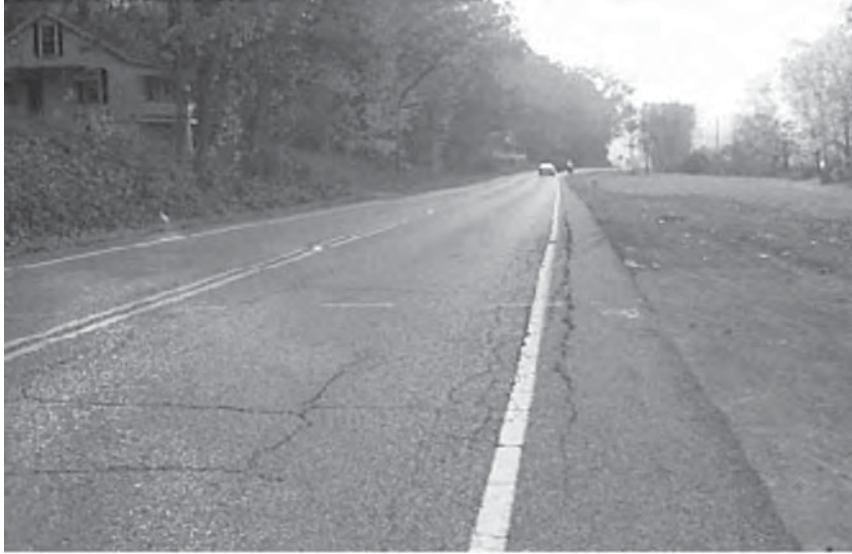
FIGURE 3.58 Localized edge cracking.
