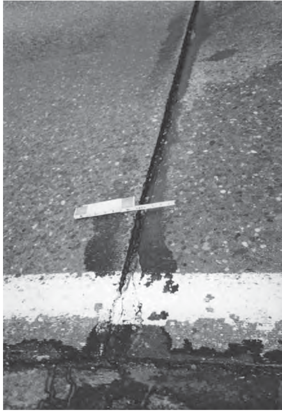
FIGURE 3.24 Example of faulting at joint in rigid pavement; pavement on right is about 1/2 in (13 mm) lower than that on left.
