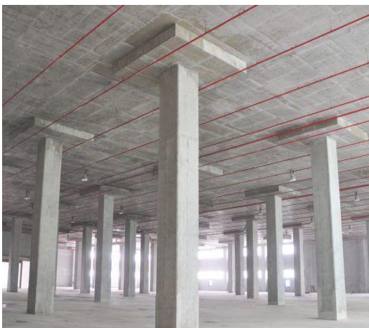
Figure 3.1: Real flat slab with drop panels
