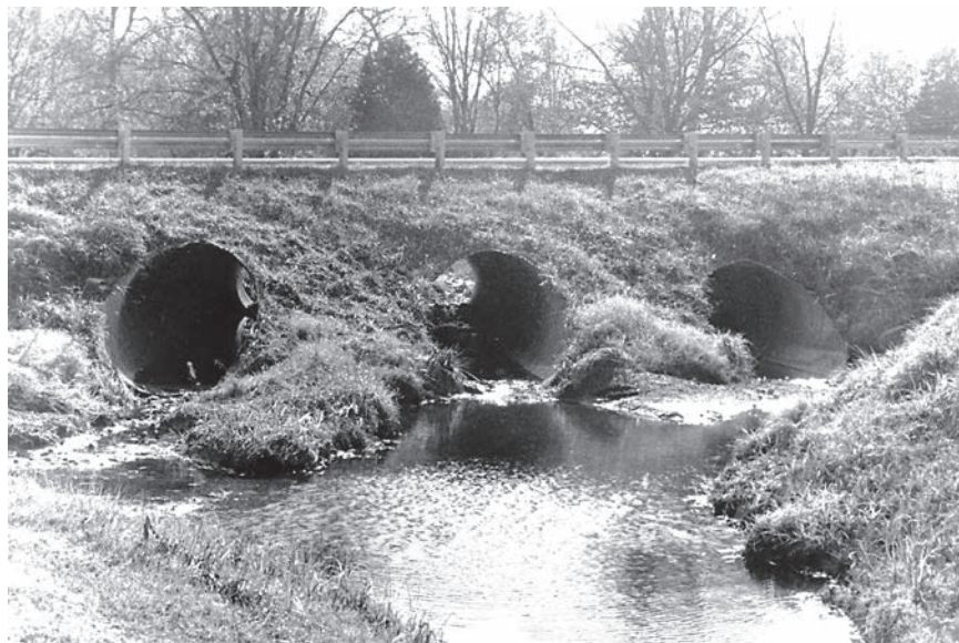
(a) Corrugated metal arch culvert (ARMCO)
