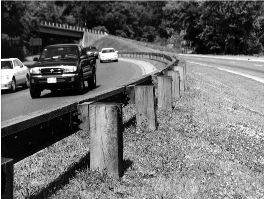
Figure 15.6 Backed Timber Guardrail
