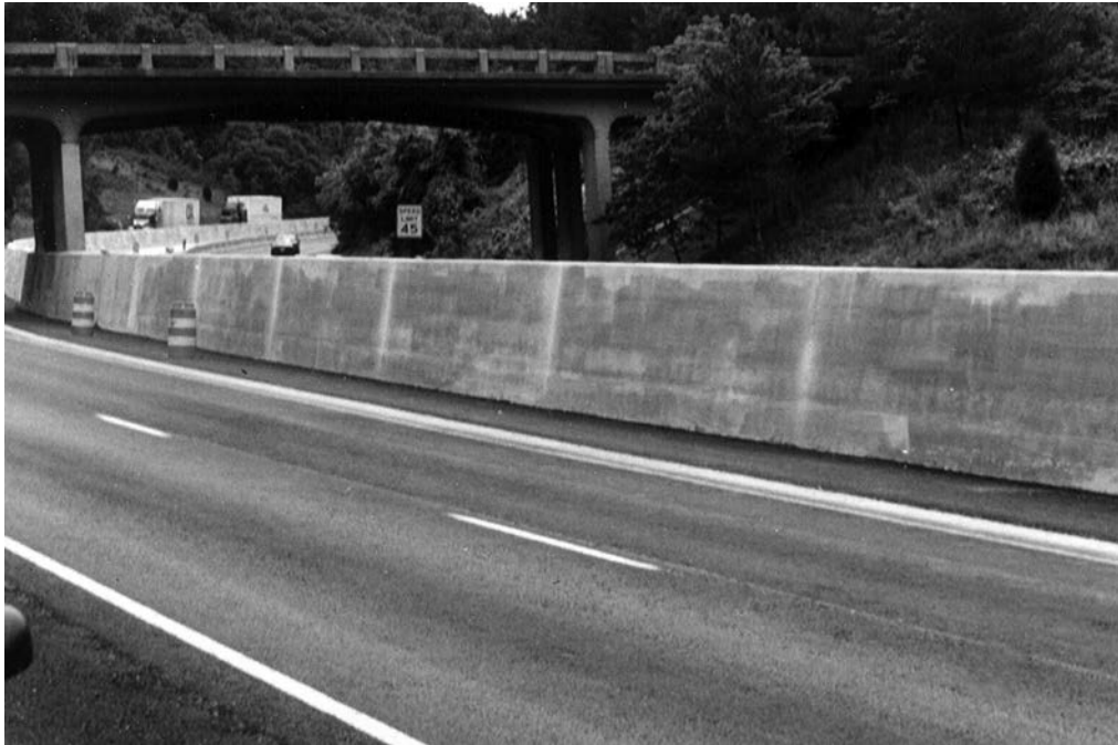
Figure 15.7 Single-Slope Concrete Median Barrier
