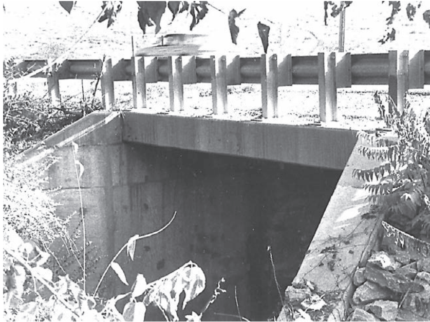
(b) Rectangular (box) culvert
