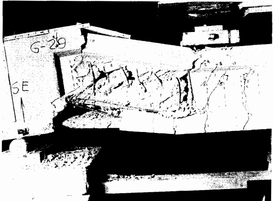
Fig. 6-24 Web crushing failure. (Photograph courtesy of J. G. MacGregor.)
