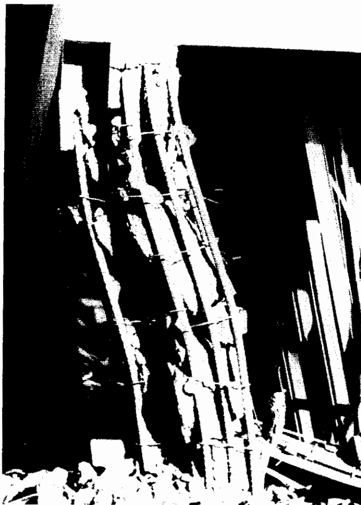
Fig. 11-6 Tied column destroyed in 1971 San Fernando earth- quake. (Photograph courtesy of National Bureau of Standards.)
