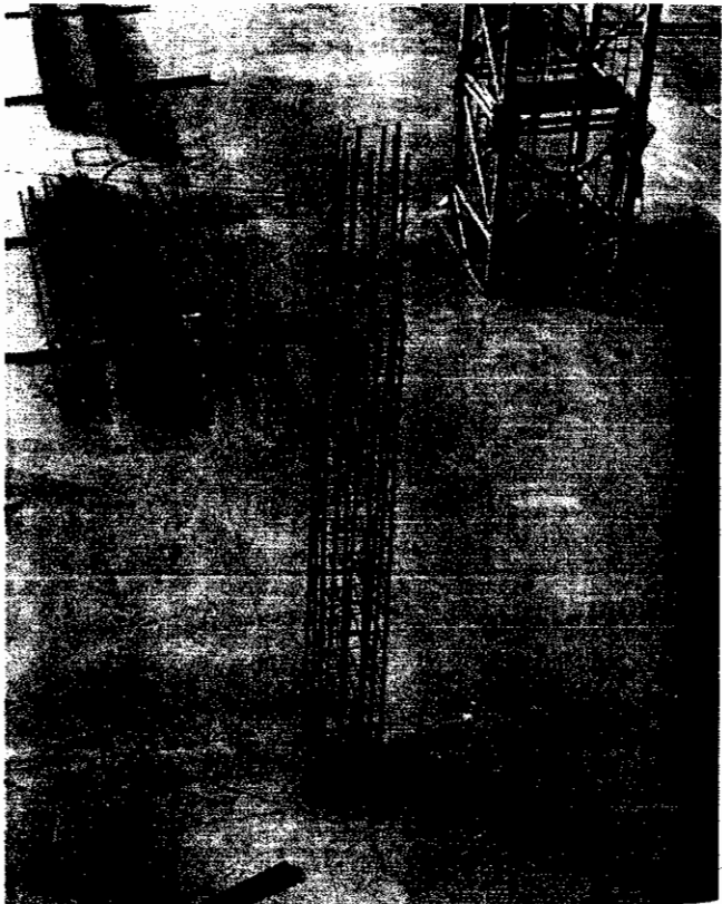
Fig. 11-2 Reinforcement cage for a tied column. (Photograph courtesy of J. G. MacGregor)
