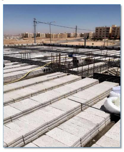
And then began reinforcing the beams with  $\phi16$  &  $\phi18$  bars according to what is in shop drawings, then cross rib, then ribs, with 2.5cm cover in all horizontal and vertical concrete sections.
