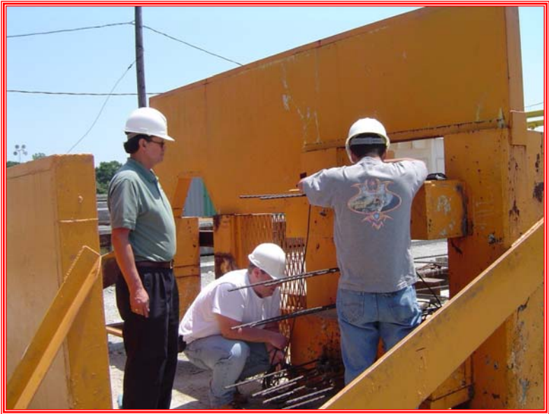
Installing Load cells at the end of the girder to measure prestress force (Dead End)
