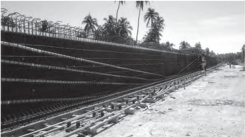
Figure 5.12 Cables in a typical beam (Photo: Benaim)
