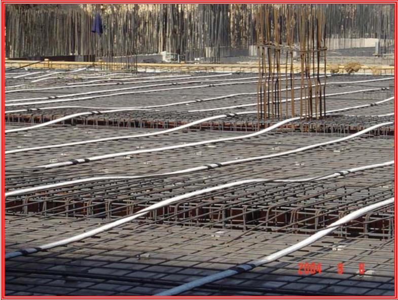
Post-Tensioned Slab
