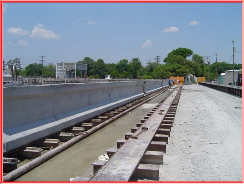
Two SCC girders and One regular
