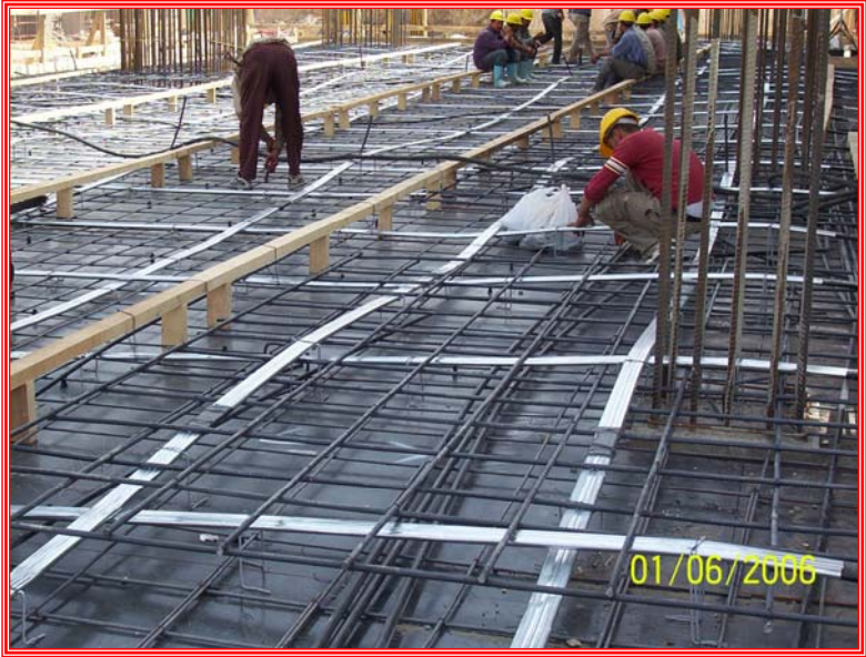
Post-Tensioned Slab
