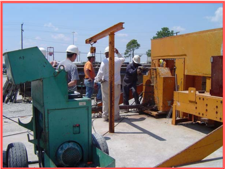
Jacking the tendons (Jacking or Live End)
