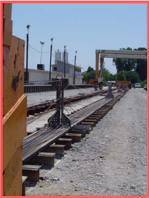
View of the tendons layout and Casting Bed
