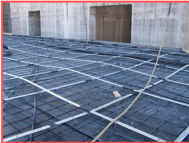
Post-Tensioned Slab
