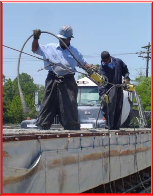
Vibrating the regular girders
