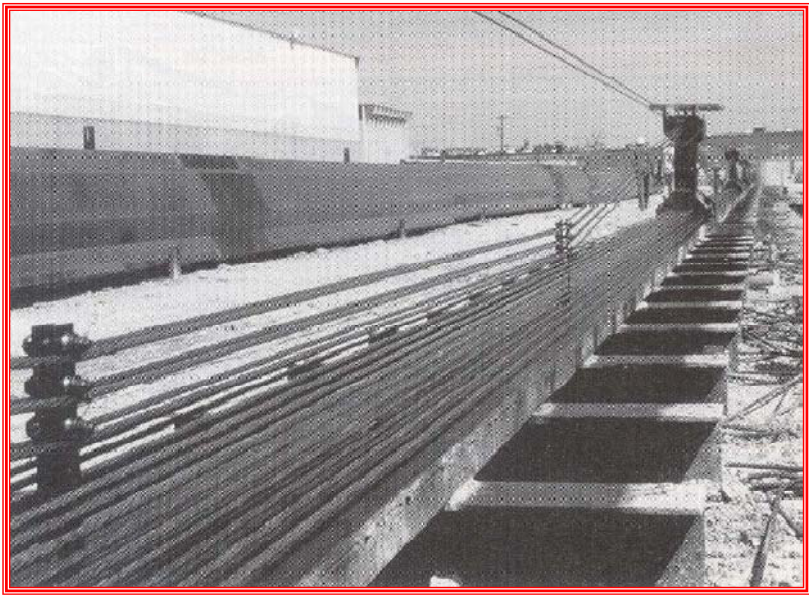
Harping of tendons in prestressing bed
