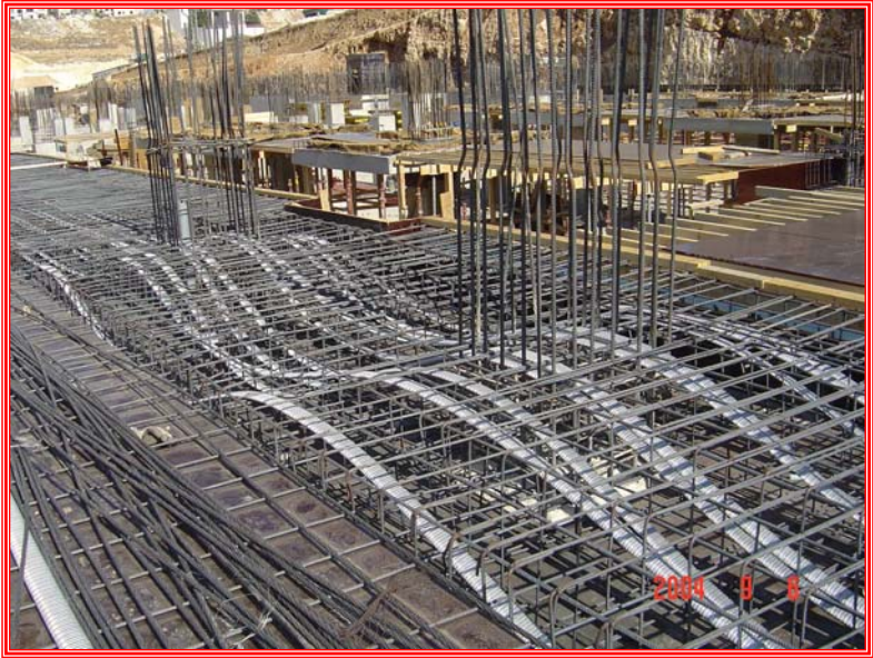
Ducts at negative moment location
