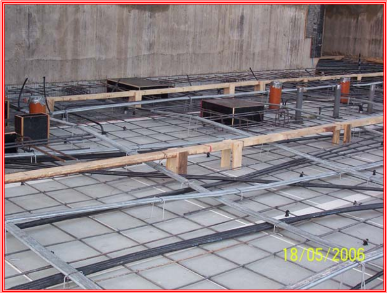
Post-Tensioned Slab
