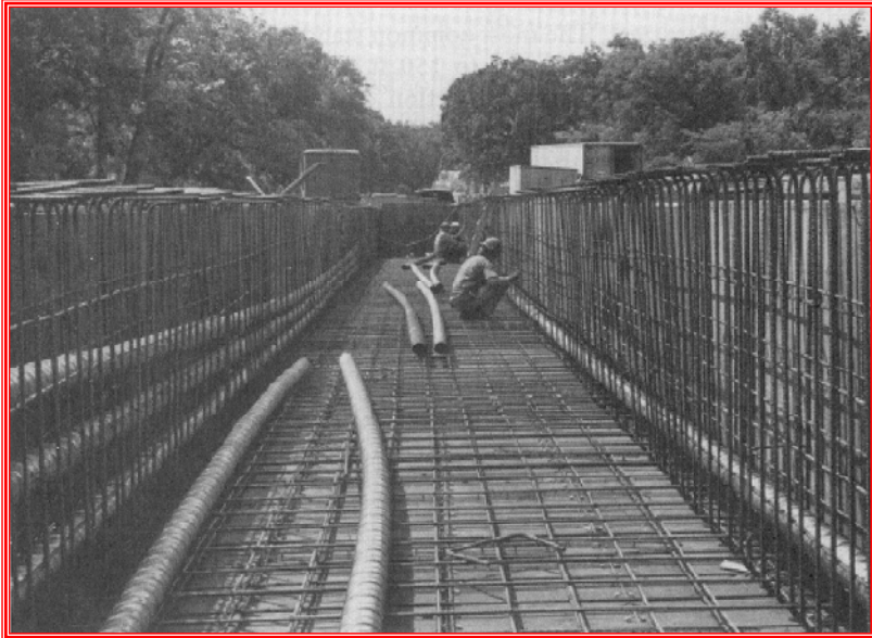
Installing Ducts
