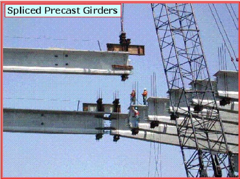
Spliced Precast Girders
