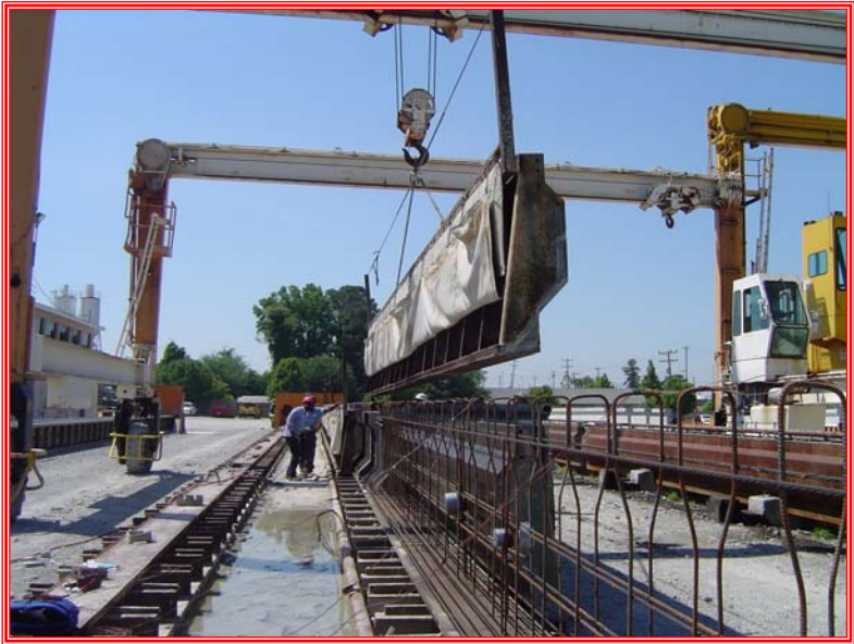
Installing forms
