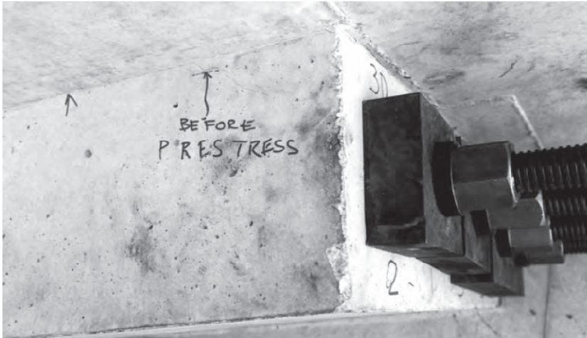
Figure 5.9d Typical prestress anchors: bar anchors (Photo: Benaim)
