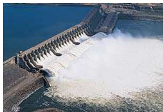
As the water falls over the dam, its potential energy is converted to kinetic energy. Use of this energy to generate electricity is called hydroelectric power.
