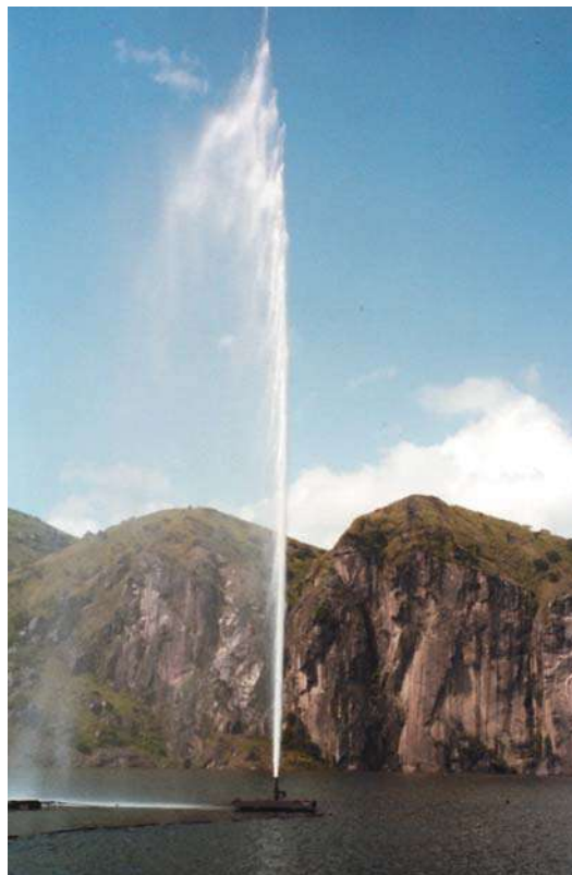
Deep waters in Lake Nyos are pumped to the surface to remove dissolved \text{CO}_2 gas.
