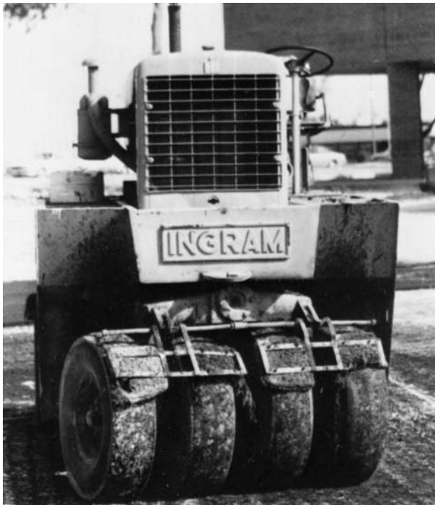
Figure 6.16 Pneumatic rubber-tired roller ( Ingram Compaction LLC )
