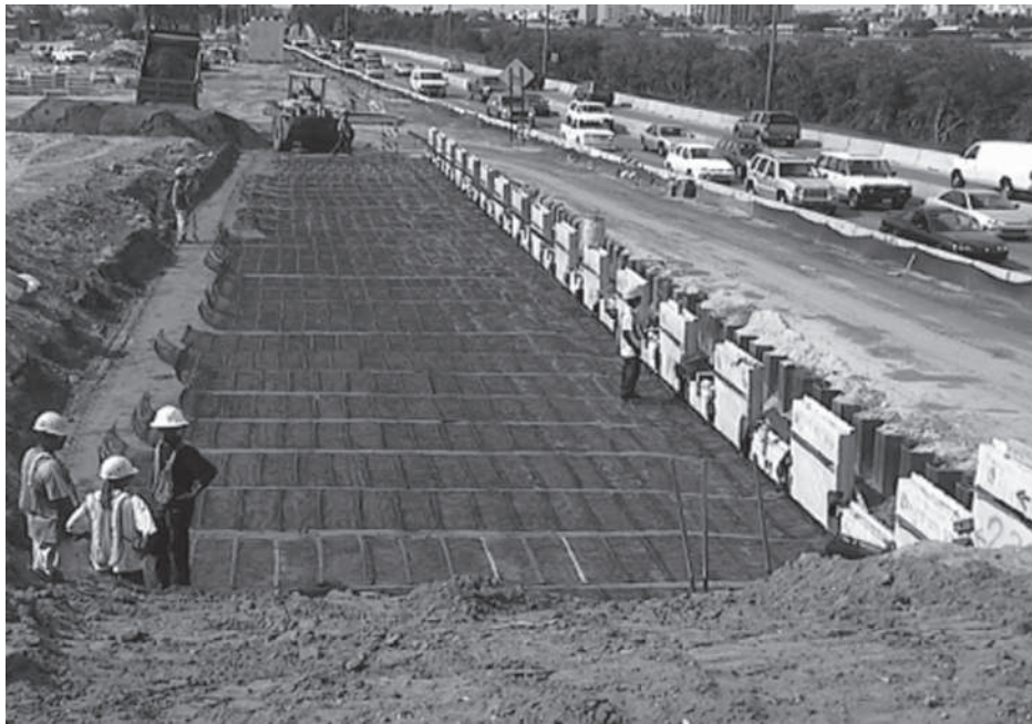
Figure 13.35 HDPE geogrid-reinforced wall with precast concrete panel facing under construction ( Courtesy of Tensar International Corporation, Atlanta, Georgia )
