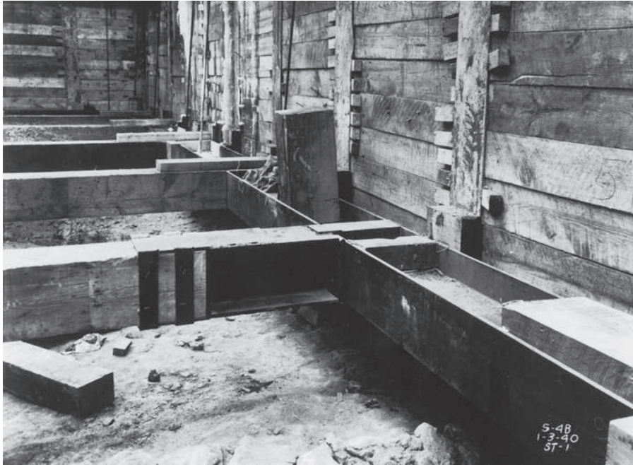
Figure 14.10 Braced cut for Chicago subway construction (Courtesy of Ralph B. Peck)
