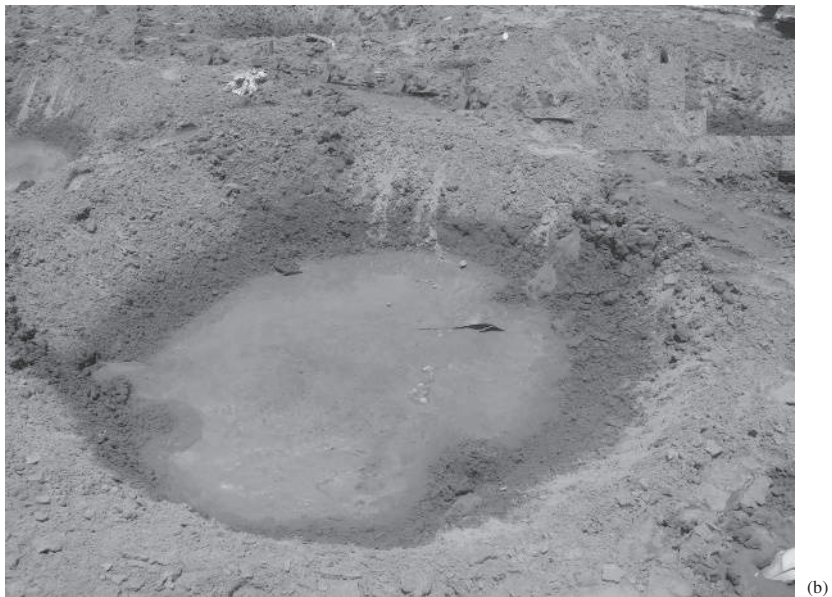
Figure 6.37 (a) Dynamic compaction in progress; (b) a site after completion of dynamic compaction (Courtesy of Khaled Sobhan, Florida Atlantic University, Boca Raton, Florida.)
