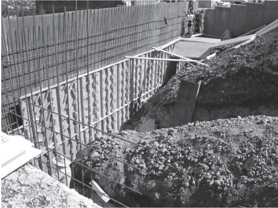
Figure 13.31 A cantilever retaining wall under construction (Courtesy of Dharma Shaky, Geotechnical Solutions, Inc., Irvine, California)
