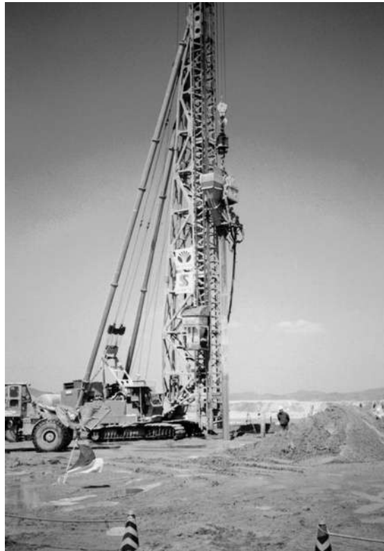
Figure 11.39 Sand drain installation in progress (Courtesy of E.C. Shin, University of Incheon, South Korea)
