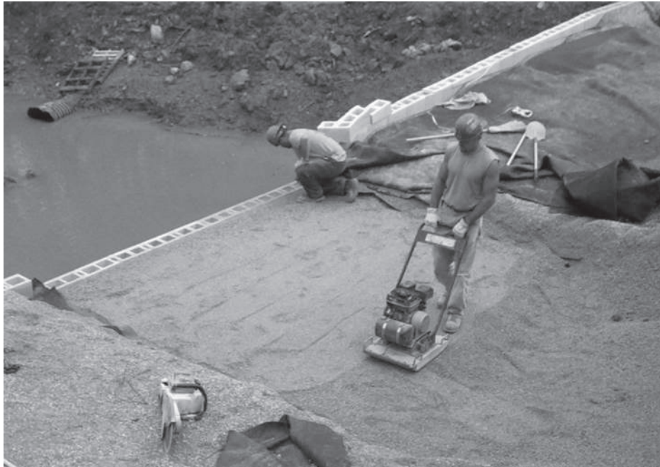
Figure 13.34 Construction of a retaining wall with geotextile reinforcement ( Courtesy of Jonathan T. H. Wu, University of Colorado at Denver, Denver, Colorado )
