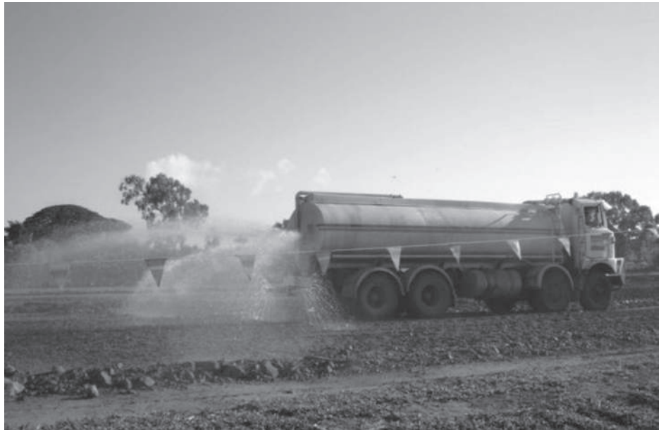
Figure 6.19 Spraying of water on each lift of soil before compaction in the field ( Courtesy of N. Sivakugan, James Cook University, Australia )
