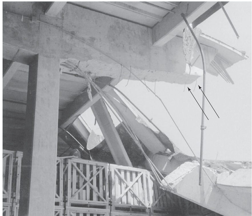
Fig. 6-2 Shear failure: U.S. Air Force warehouse. Note the small size and large spacing of the vertical web reinforcement that has fractured. (Photograph cour- tesy of C. P. Siess.)
