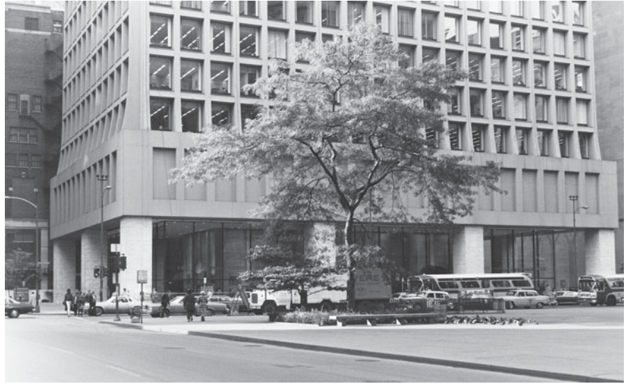
Fig. 17-26 Three-span deep beam, Brunswick building, Chicago. (Photograph courtesy of J. G. MacGregor.)
